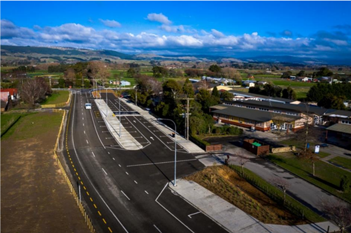
Figure 3 - Stoney Creek Road Safety Upgrade Project
