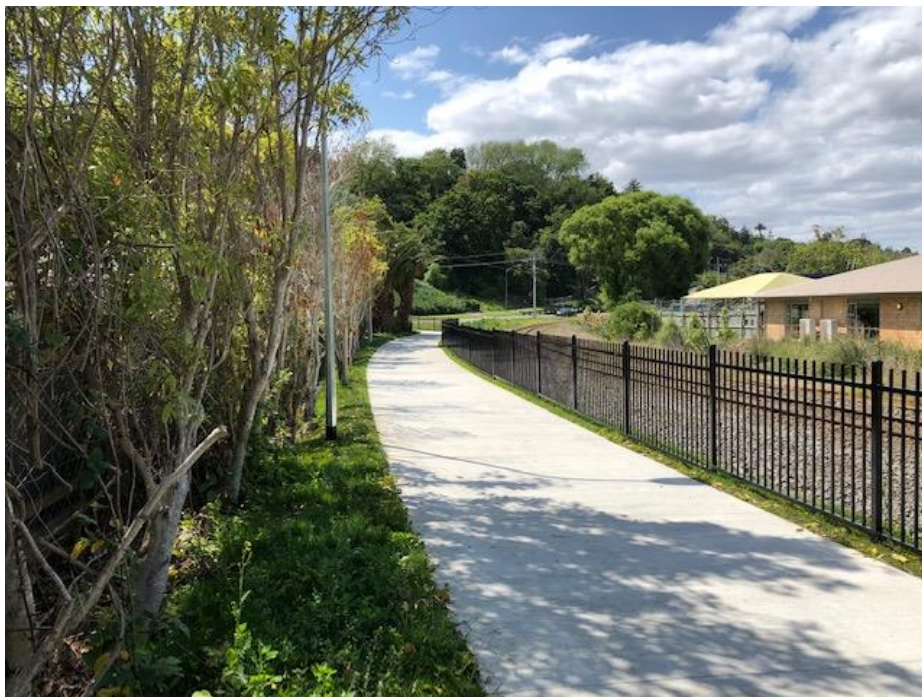
Photo: Completed Te Tuaiwi shared pathway located in Kiwirail corridor between Glasgow Street and SH3.
