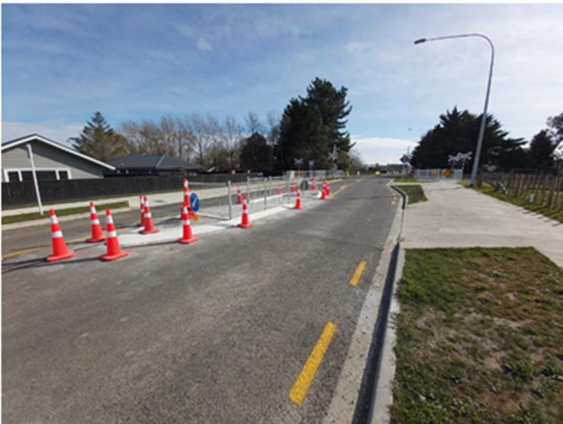
Figure 2 - James Line Pedestrian Refuge
