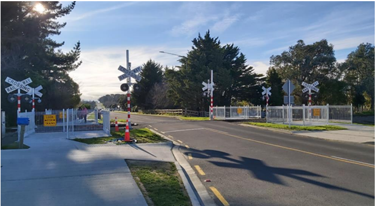
Figure 1 James Line – Railway Crossing Safety Upgrade
